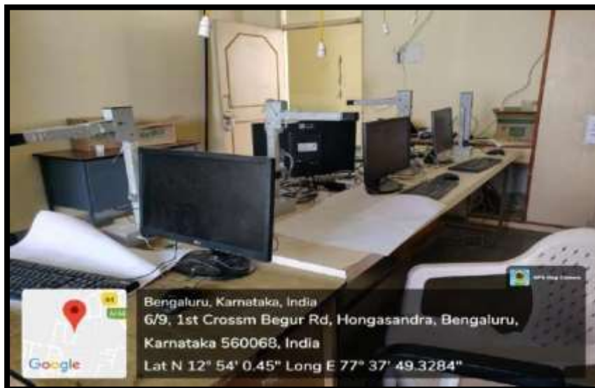
Strong Room with Access Control
